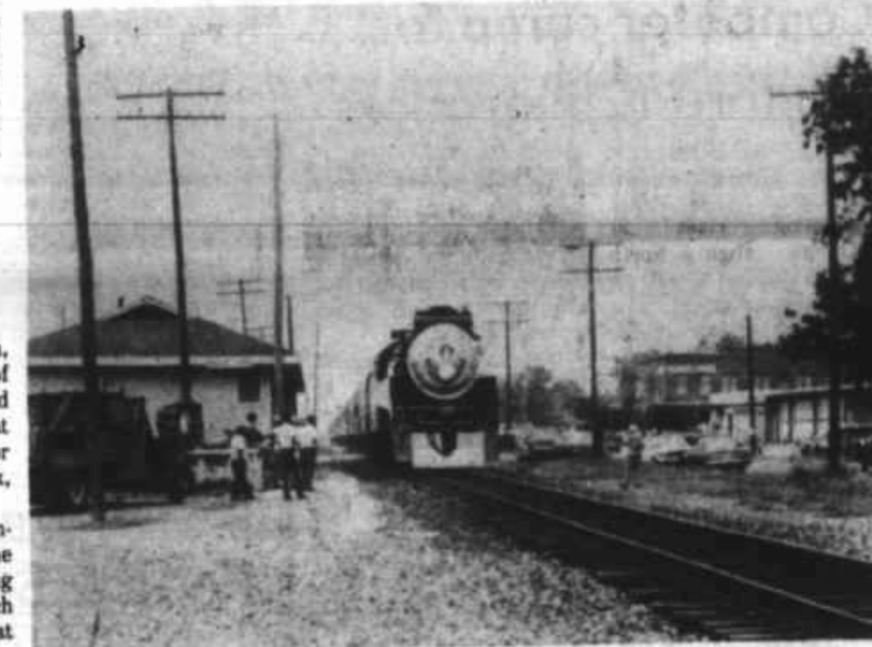
The SP steam engine made tracks through Eagle Lake last Thursday about 12:35 p.m. The engine, restored in traditional colors of red, orange and black, lead an assortment of equipment enroute to New Orleans. It will be on display at the 1984 World's Fair there.
